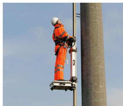
The system offers its user multiple safety features through a firmly fixed connection to a rail. The connection of the climbing devices to the rail ensures to climb safely whilst making missteps or falls nearly impossible. The rail can solely be climbed by using a climbing device and therefore prevents any unauthorized access.
