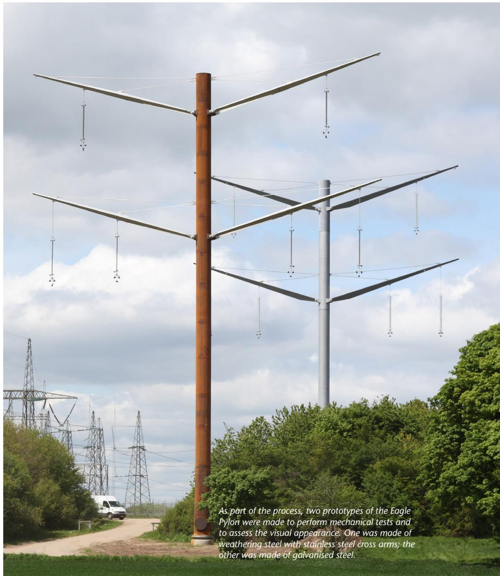
*As part of the process, two prototypes of the Eagle Pylon were made to perform mechanical tests and to assess the visual appearance. One was made of weathering steel with stainless steel cross arms; the other was made of galvanised steel.*
